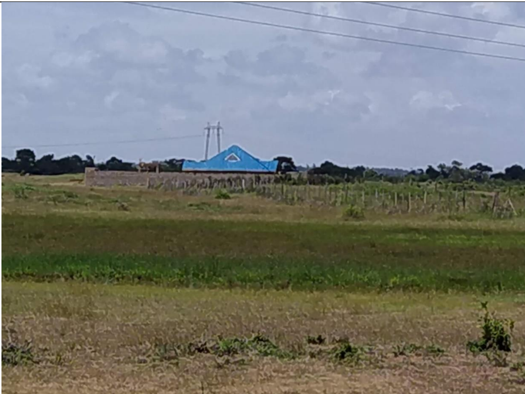
A NEW HOUSE WITH BLUE ROOFTOPS BEING CONSTRUCTED
